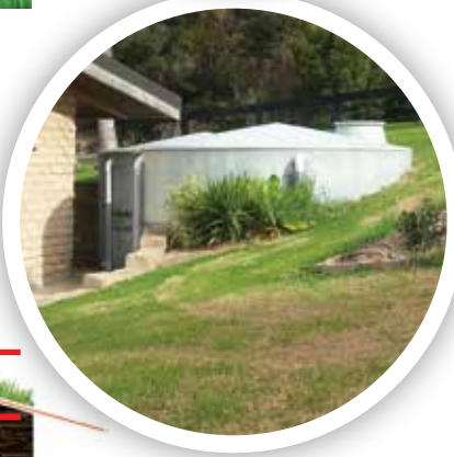
Standard 25,000L Tank Unequally Buried
